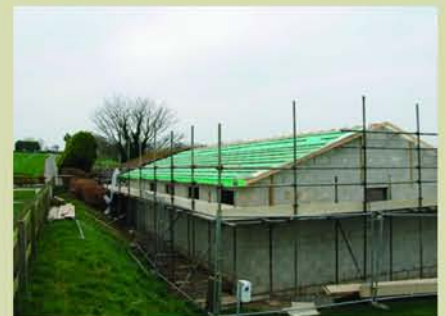
Construction to date 15/12/2007
